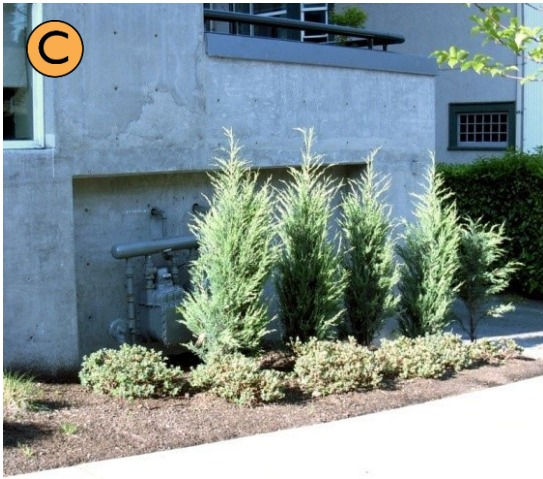
Figure 15.96.110.D Utility meter location and screening - good and bad examples.
