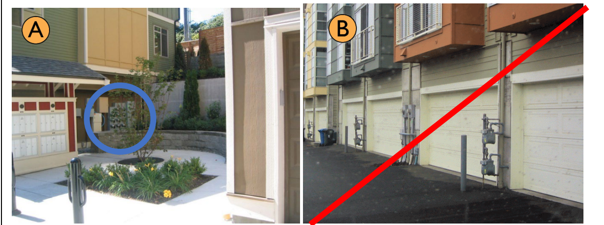
Figure 15.96.110.D Utility meter location and screening - good and bad examples.
