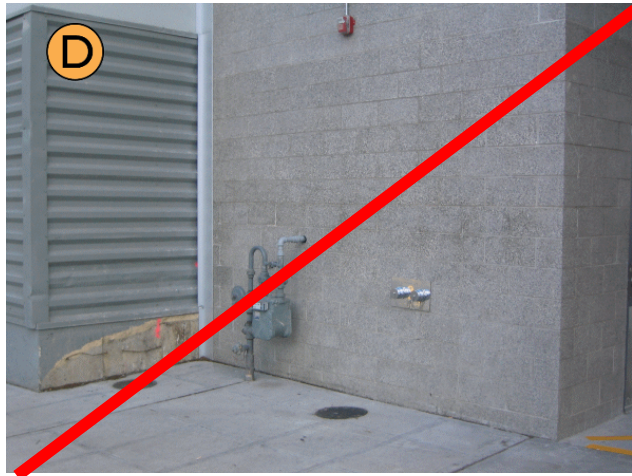
Figure 15.96.110.D Utility meter location and screening - good and bad examples.
